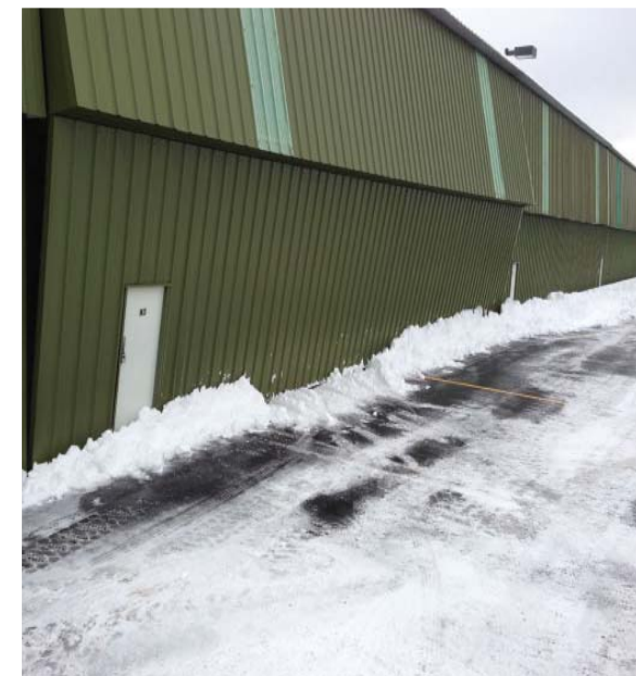
A hangar door improperly closed over uncleared snow and ice.
