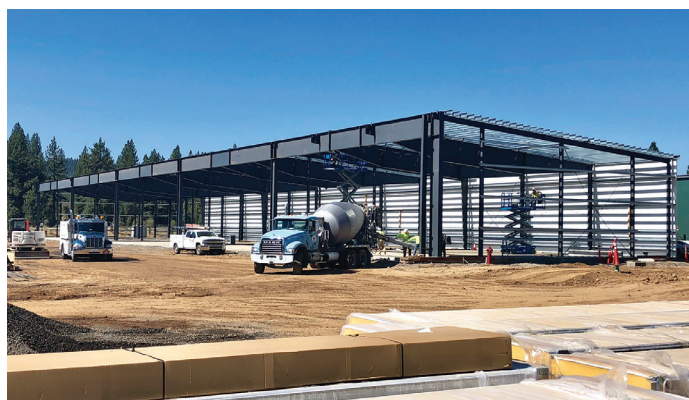
Hangar Row November under construction summer 2018.
