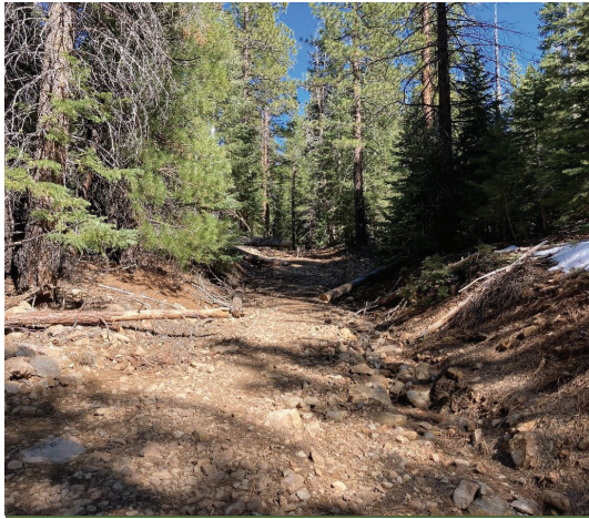
▲ An abandoned logging road with significant erosion.
