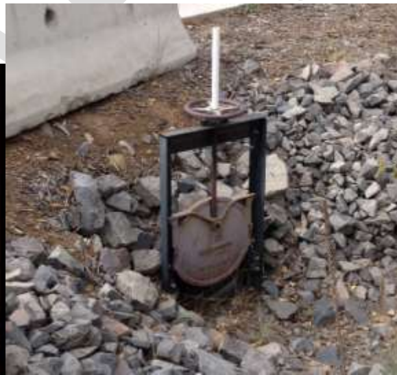
Storm Drain Pipe and Slide Gate
