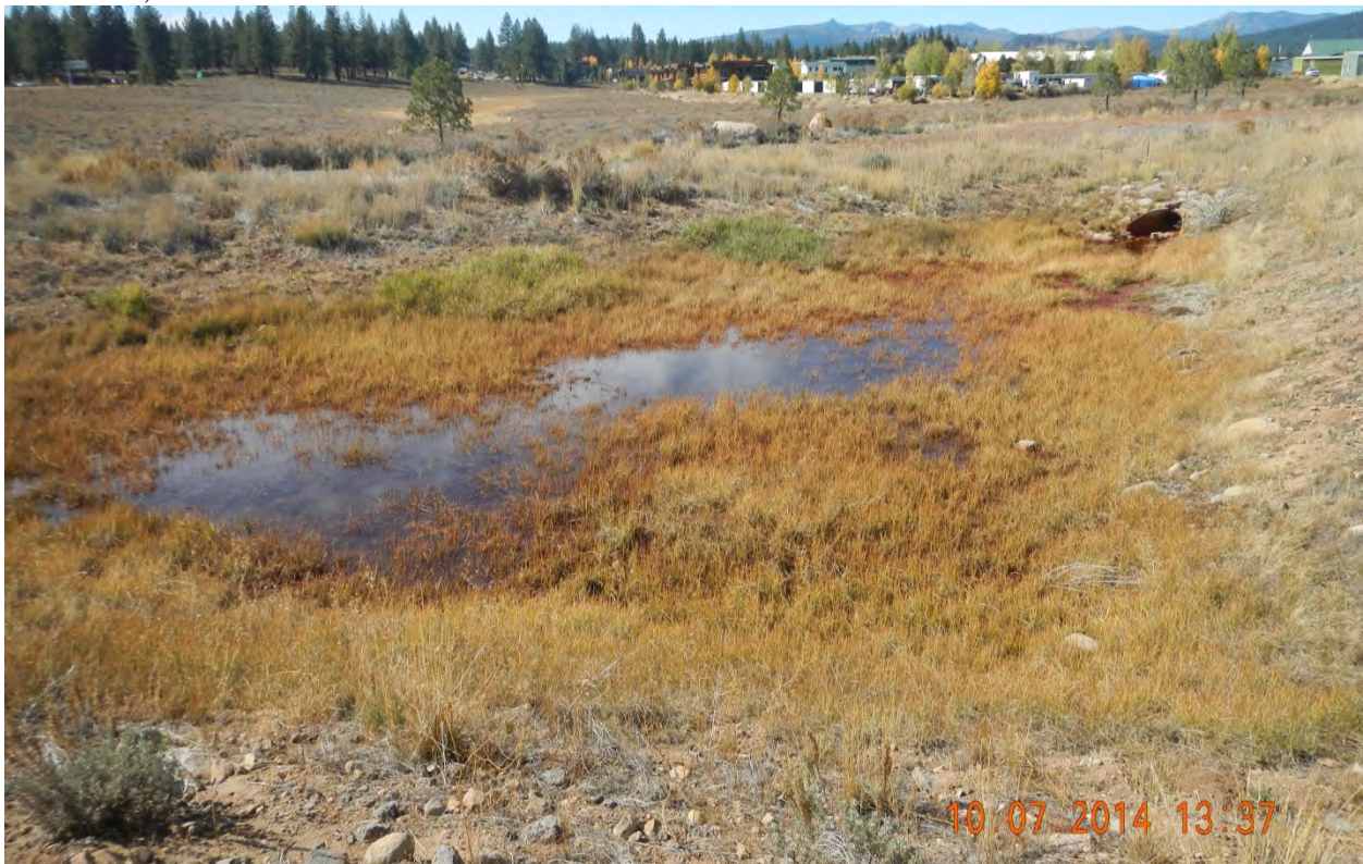
Photo 6. Detention basin with standing water. Facing approximately west. October 7, 2014.
