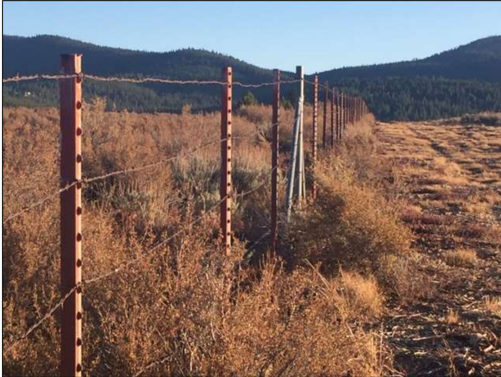
Photo 5: View of the airport perimeter fence along Martis Dam Road.
