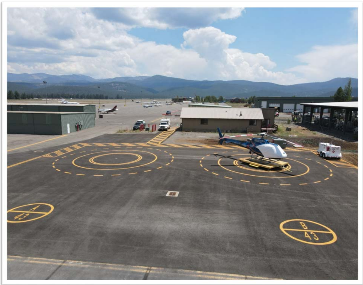
New Emergency Medivac Facility Constructed Summer of 2020.
