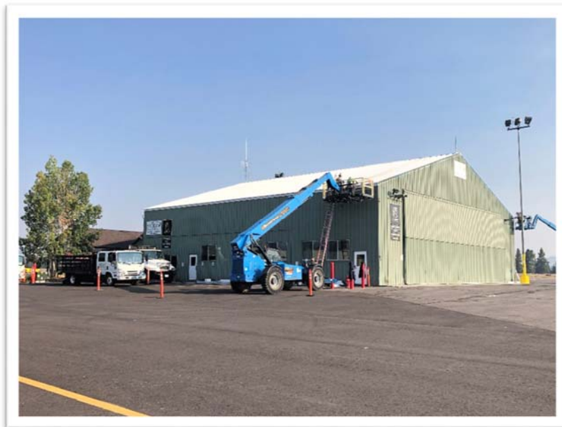
New Roof Installation on Hangar 1 in Summer 2020
