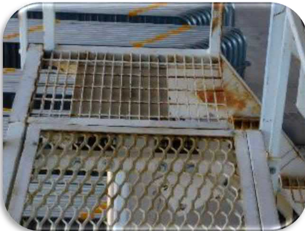
Figure 5-41 shows the general condition of the stairway support structure and grating.
