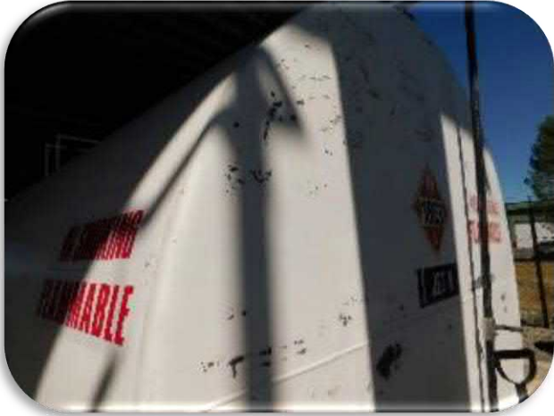
Figure 5-39 shows the condition on the back ends of the tanks. Note the numerous delaminations.
