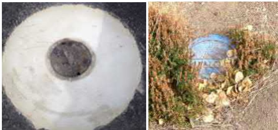
Figure 9-3. Water System Valves
