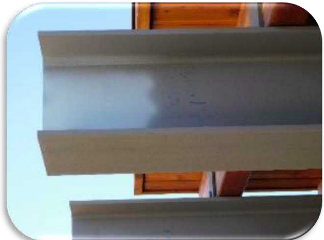
Figure 5-23 shows an example of the condition of the wood surfaces.
