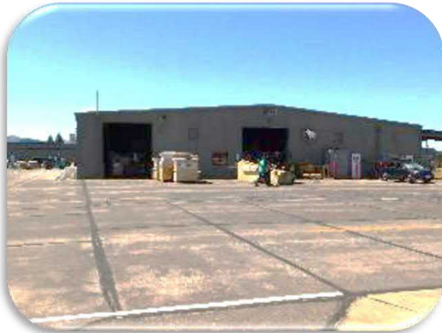
Figure 5-50 shows a general view of the warehouse.
