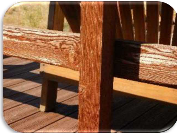
Figure 5-33 shows the general condition of the wood decking and railings.
