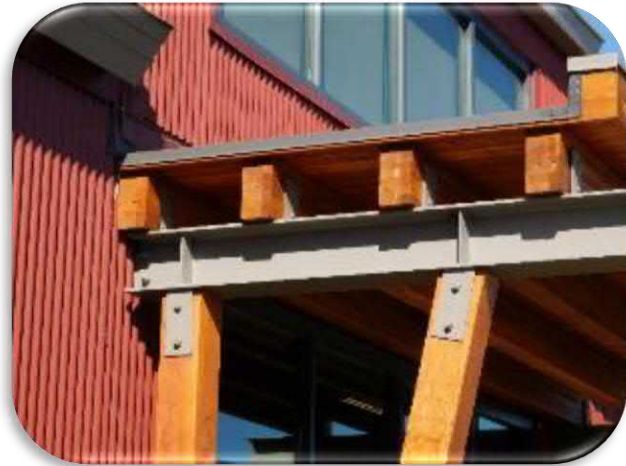
Figure 5-24 shows a structural member with the markings visible through the coating.
