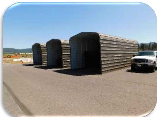
Figure 5-26 shows a general view of the sheds located adjacent to the maintenance facility.
