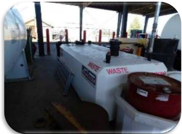
Figure 5-48 shows a general view of the concrete waste tank
