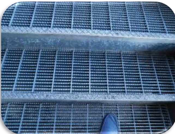
Figure 5-10 shows a general view of the galvanized steel decking.
