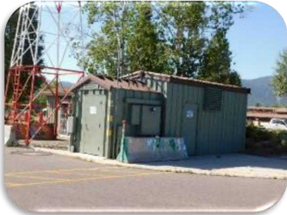
Figure 5-14 shows a general view of the generator building.
