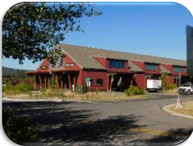
Figure 5-22 shows a general view of the WOB
