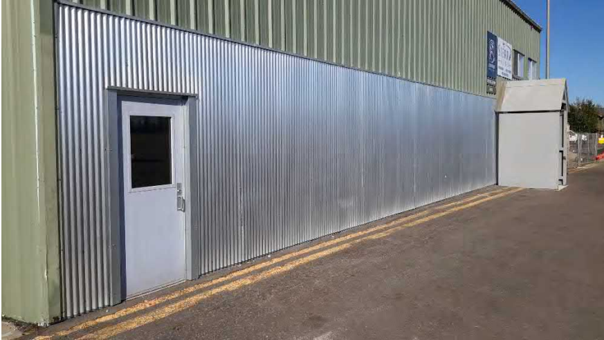
Figure 7 Building 1 - new furred panel area, north wall
