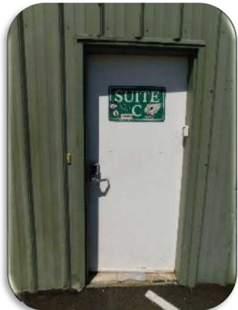
Figure 5-49 shows an example of the condition of the coating on the doors (bright and glossy). Note, however, that the adjacent siding is faded and flat.
