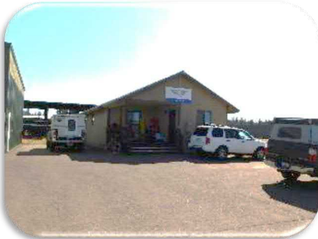
Figure 5-31 shows a general view of the West Side Modular.
