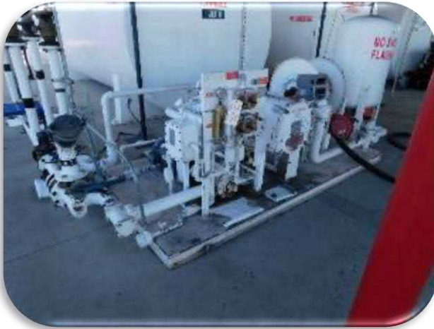
Figure 5-43 shows a general view of some of the painted surfaces on the pumping station.
