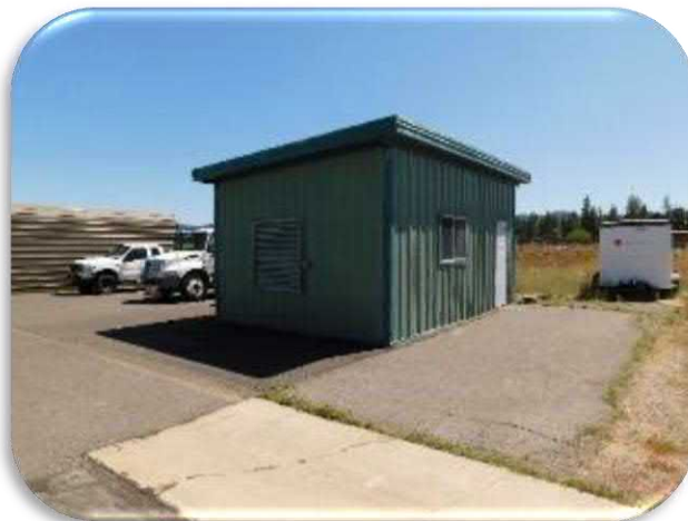
Figure 5-16 shows a general view of the generator building shed.
