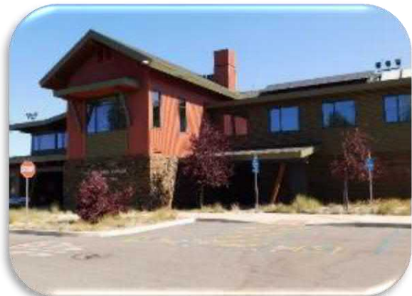
Figure 5-5 shows a general view of the Truckee Tahoe Airport Administration Building.
