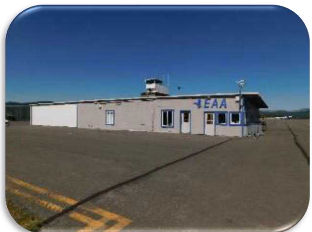
Figure 5-56 shows a general view of the EAA Building.
