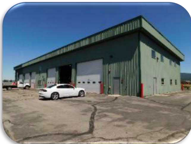
Figure 5-25 a general view of the maintenance facility
