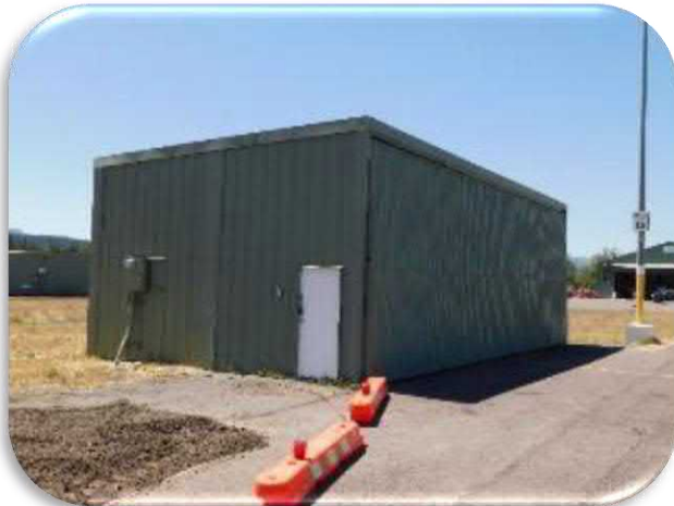
Figure 5-54 shows a general view of the Phoenix.
