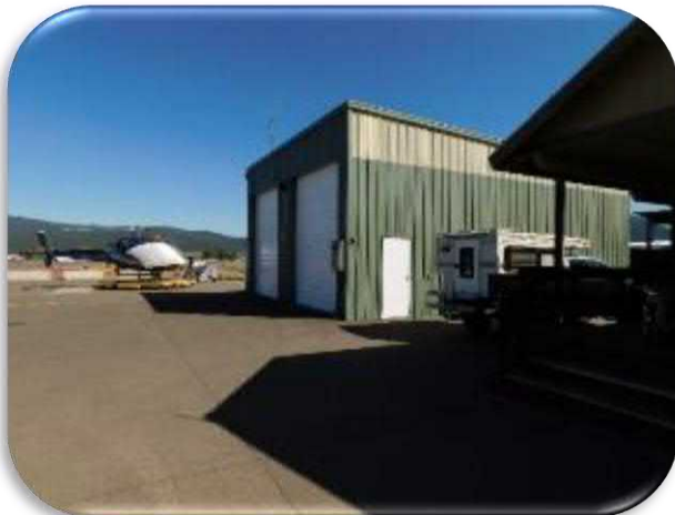
Figure 5-29 shows a general view of the garage.
