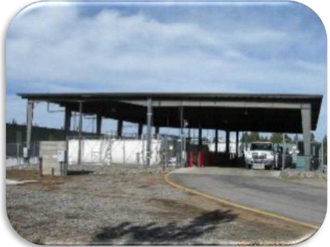
Figure 5-34 shows a general view of the Fuel Farm.
