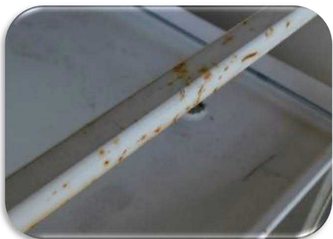
Figure 5-42 shows the typical condition of the stairway handrails.
