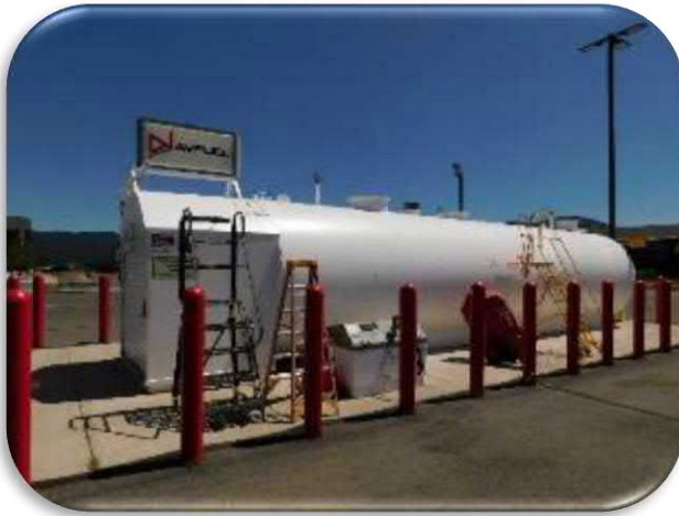
Figure 5-17 shows a general view of the self-serve tank.
