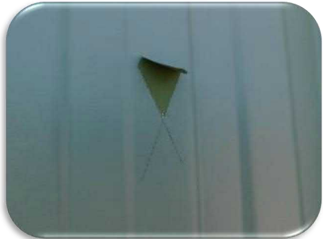
Figure 5-72 shows an example of an adhesion test indicating poor coating adhesion.
