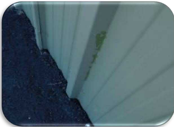
Figure 5-67 shows an example of one of the infrequent delaminations on Hangar C.
