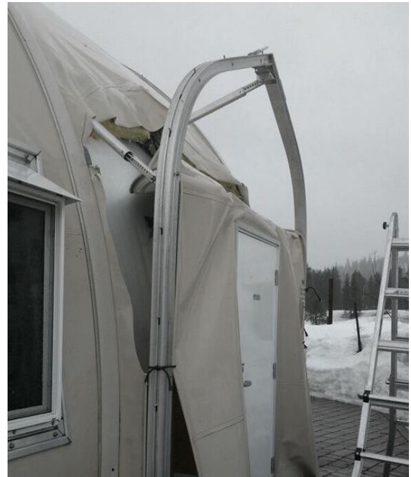
Museum structural damage during 2017 storms
