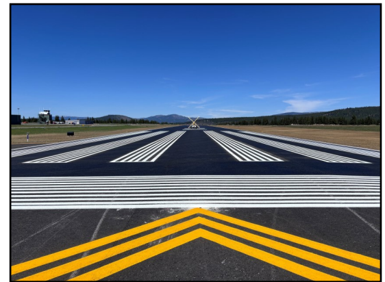
New pavement and fresh paint on Runway 2
