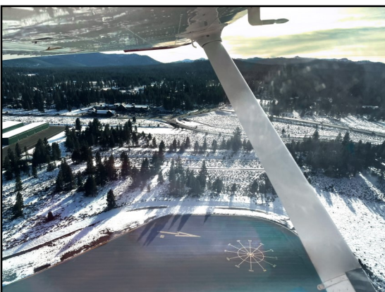
11 Runup area markings guide pilots to bypass bridge
