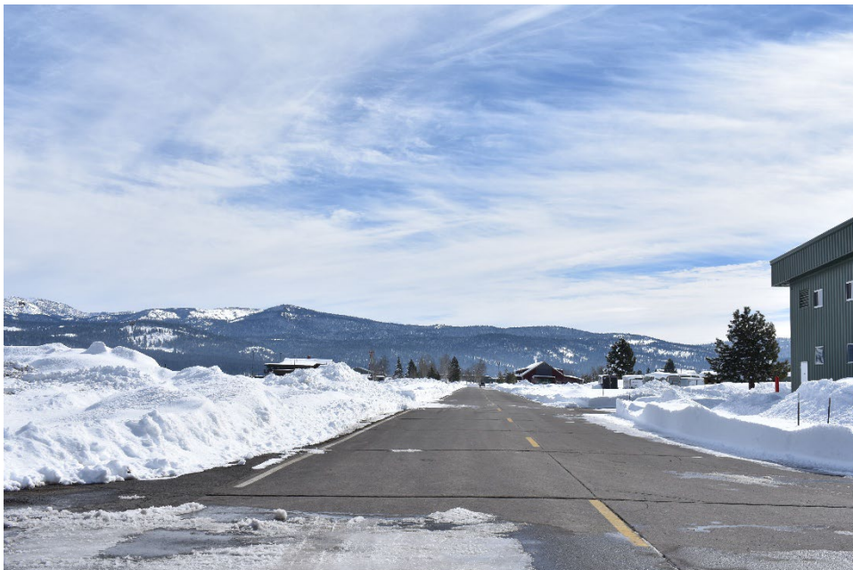
VIEW LOOKING EAST TOWARD CHANDELLEY WAY AT ITS INTERSECTION WITH AVIATION WAY
