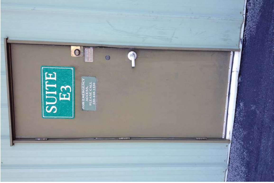
PHOTOS OF TYPICAL TENANT SPACE ENTRY DOORS. NON-ACCESSIBLE DUE SILLS AND THRESHOLDS THAT DO NOT MEET THE ACCESSIBILITY REQUIREMENTS.
