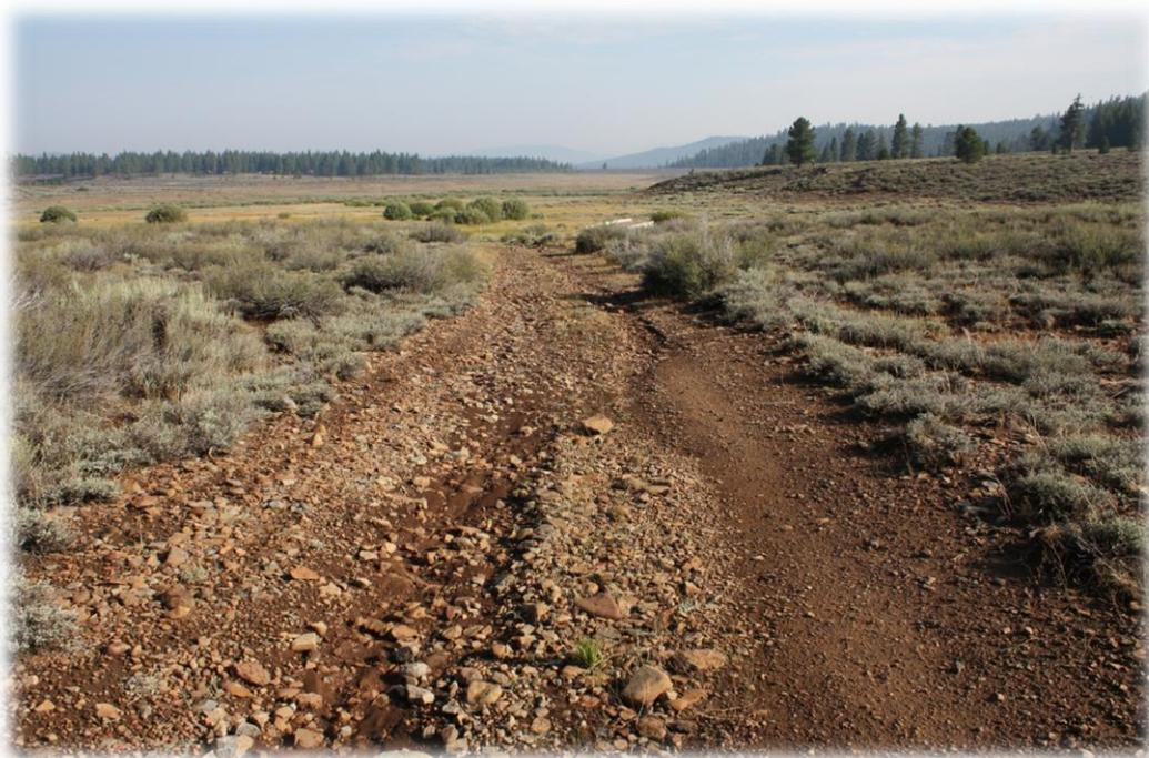
Picture 1: Surface erosion on Waddle Ranch main access road following an August 2012 summer rain storm. Surface soils eroded in such circumstance are transported to East Martis Creek.
