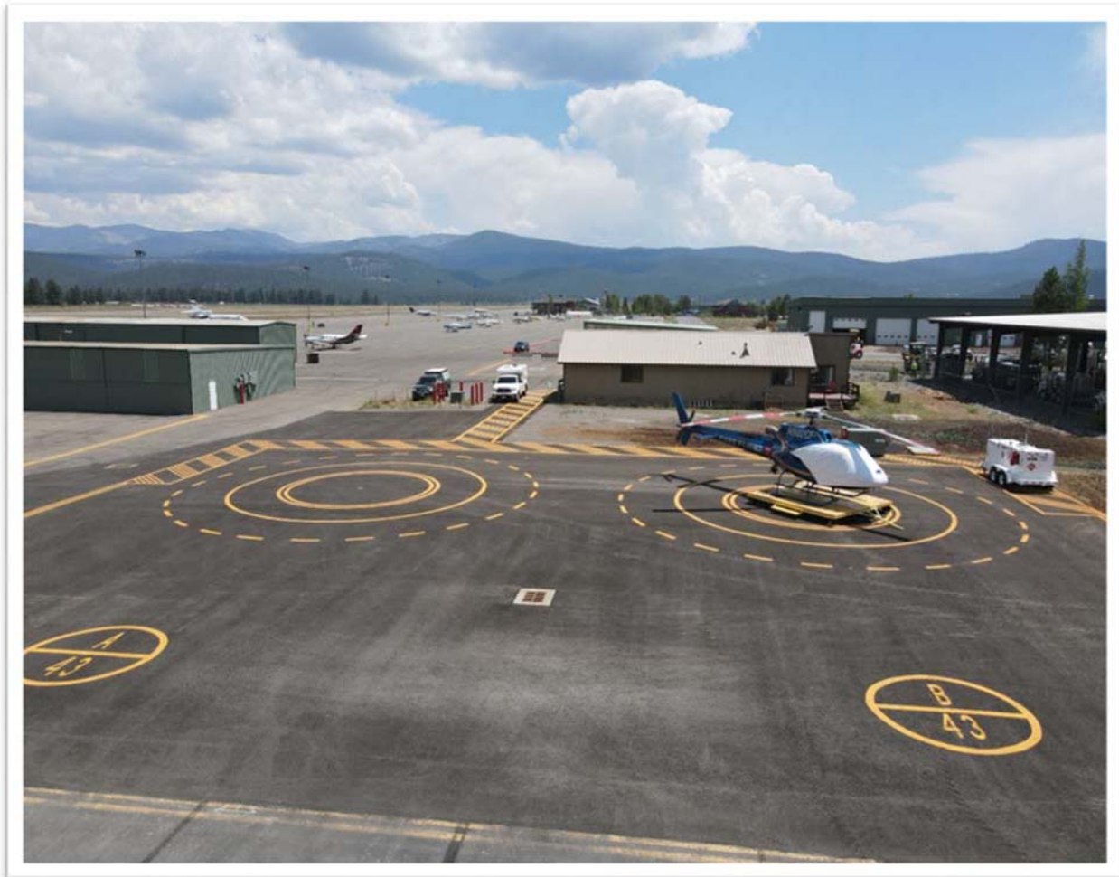
New Emergency Medivac Facility Constructed Summer of 2020.
