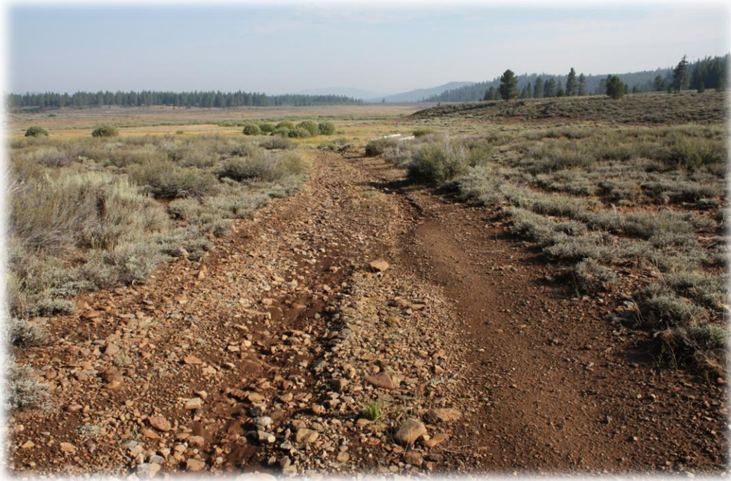
Figure 1: Rilling on the Waddle Ranch main access road following an August 2012 rainstorm.
