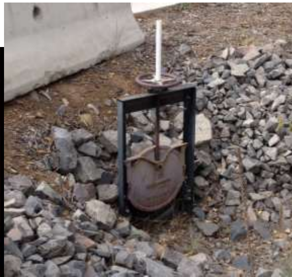
Storm Drain Pipe and Slide Gate
