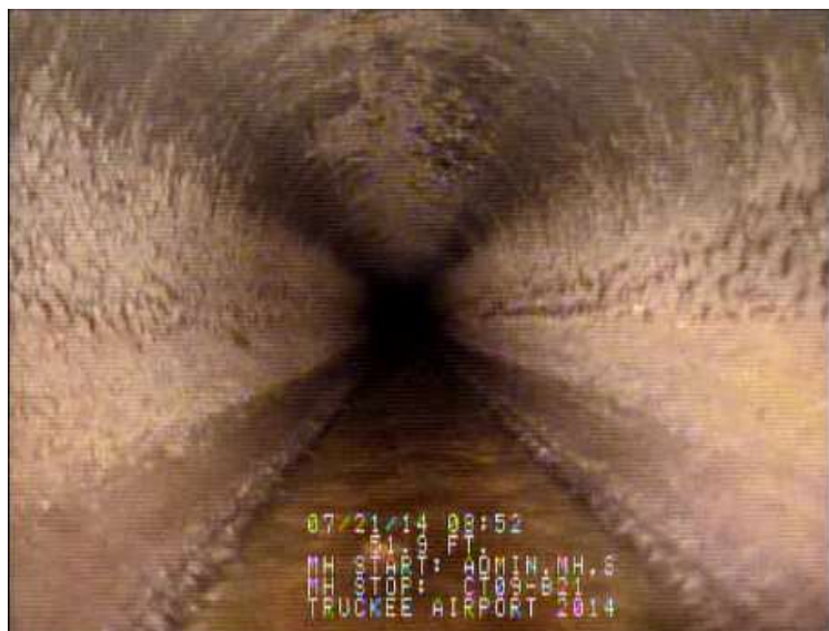
Interior of sanitary sewer pipe serving Administration Building
