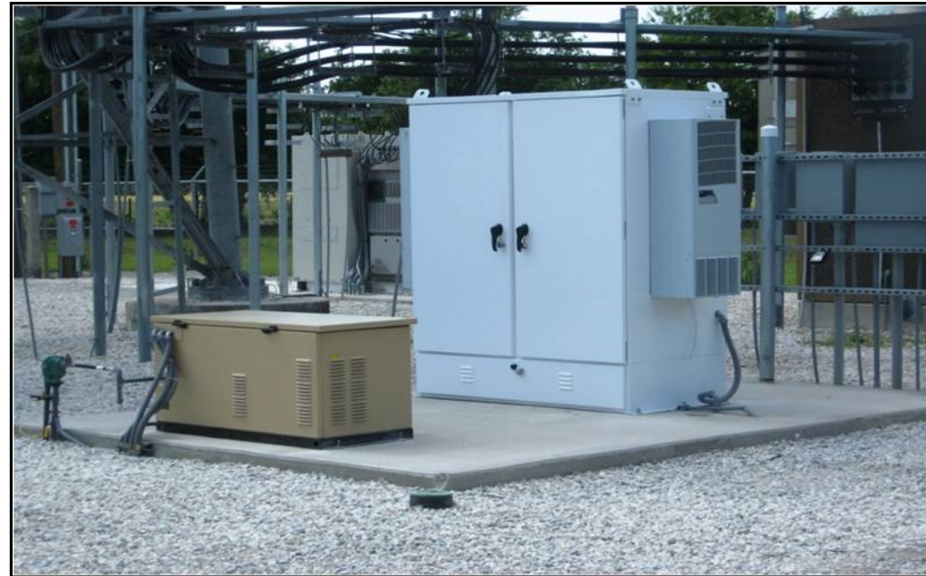
Radio Station Equipment Cabinet & Generator
