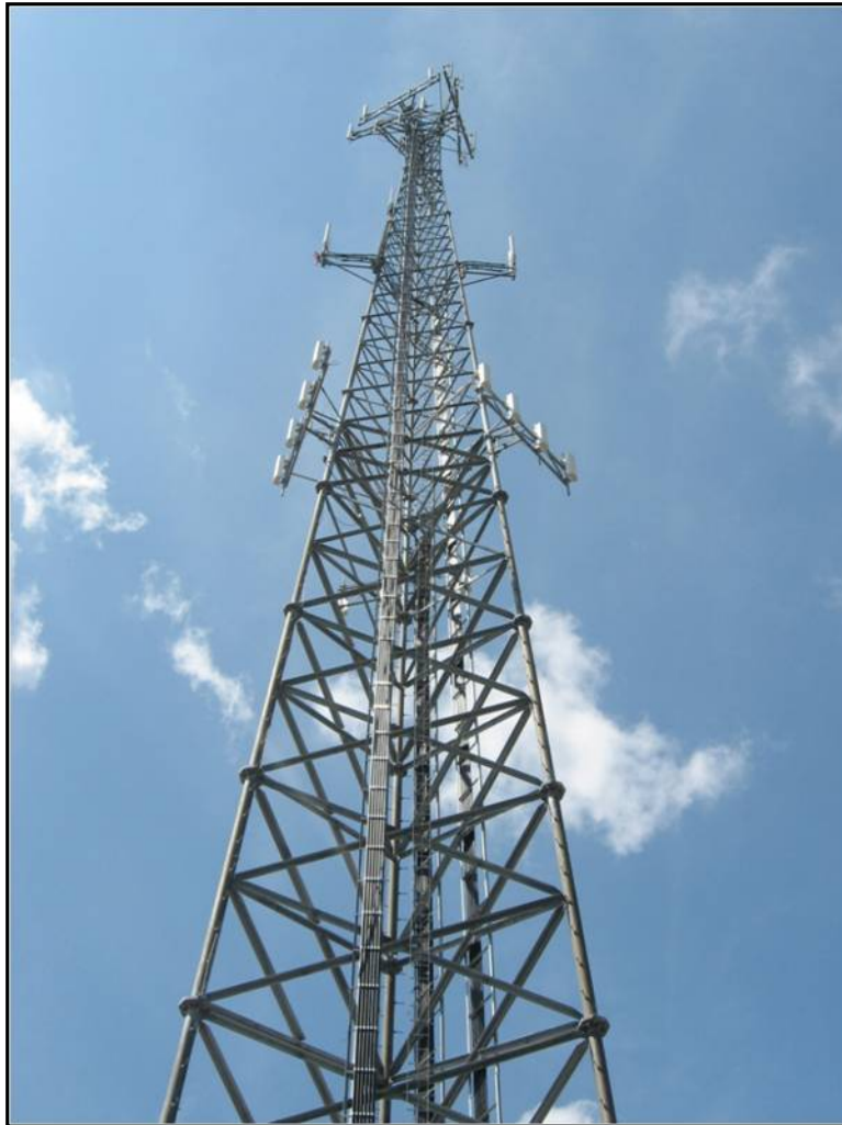
Antenna Array – 1090, UAT, GPS
