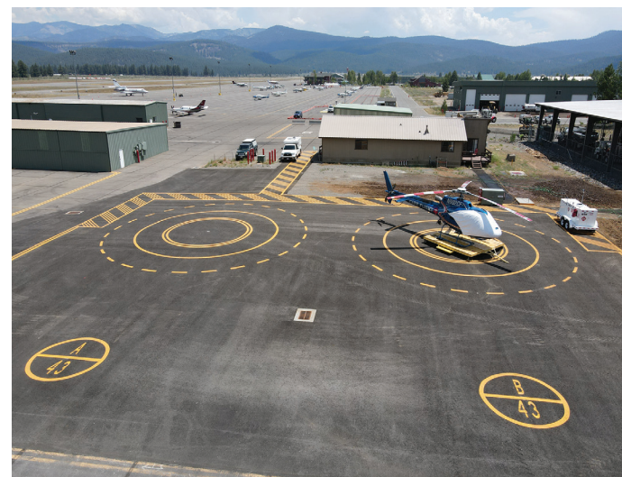
A bird's-eye view of the completed Heliport on the west side of the airfield.
